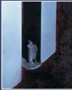
Bottom Mount is the lower pin inserted through a bearing washer into a 1/2" x 2" hole drilled into the floor
